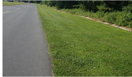
Vegetative Filter Strip
