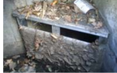
Connector Pipe Screen
