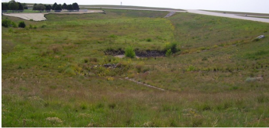
Surface Detention Basin
